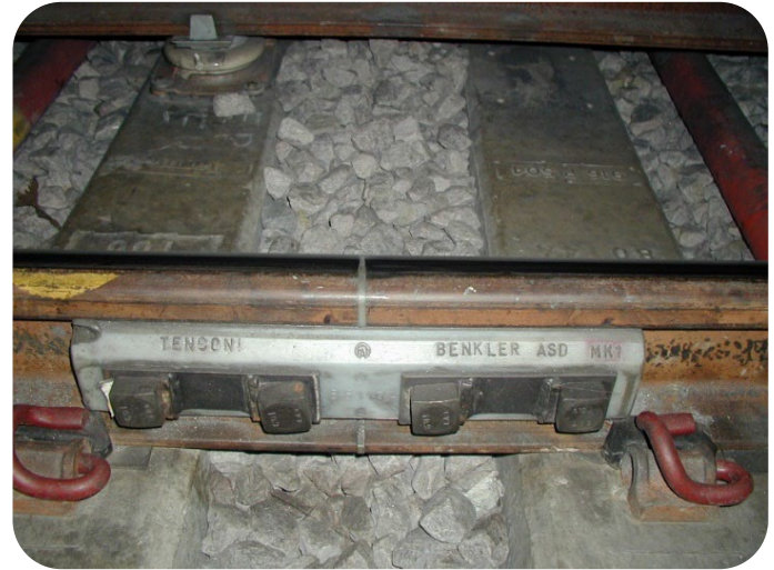
Insulated Rail Joints
